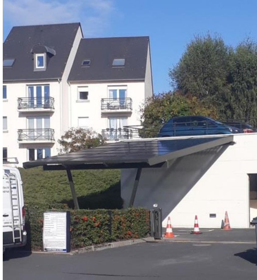
Ombrière de parking – 2 places
