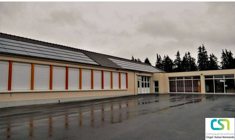
Installation Photovoltaïque de 36 kWc
